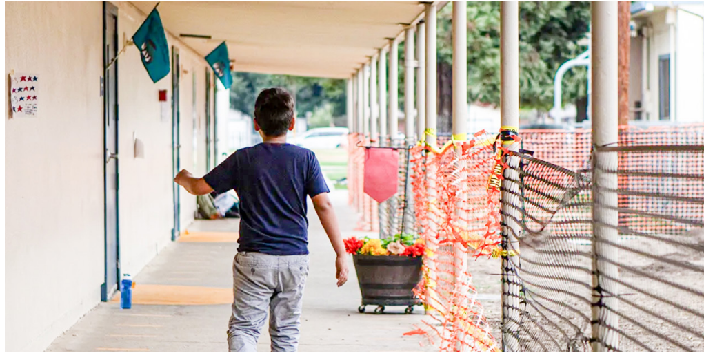
Construction sites in the hallways of Keyes Elementary School in Keyes on Nov. 15, 2023.
