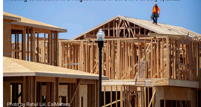
Housing construction in a neighborhood in Elk Grove on July 8, 2022.
